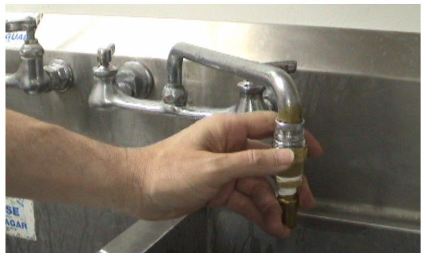
Connect the Auto-Fill Water Supply Hose to a faucet and turn on the water
